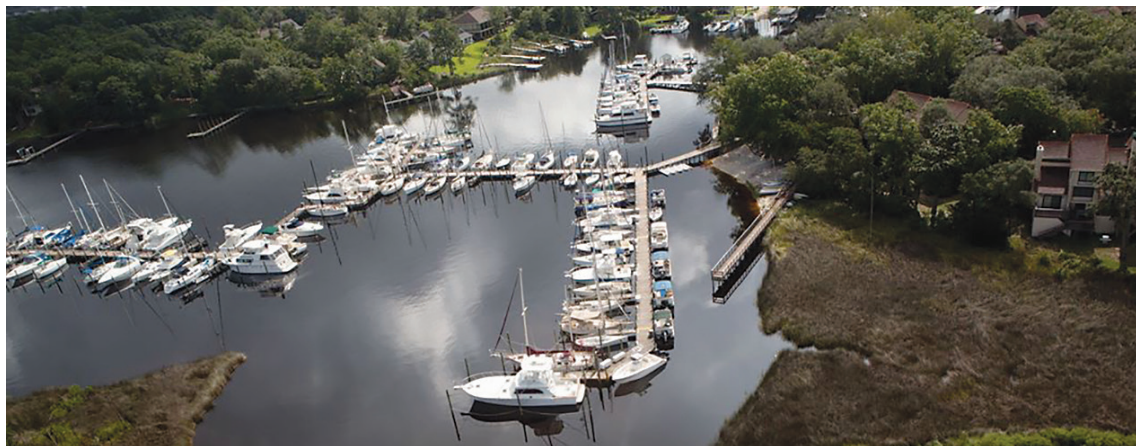
The Bluewater Marina has 120 slips and a storage facility for 200 boats.
