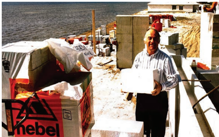
Raimund Herden is pictured in 1993 holding an aerated concrete block. The lightweight alternative to concrete manufactured by a German company, was used in Bluewater Bay for the first time in North America.
